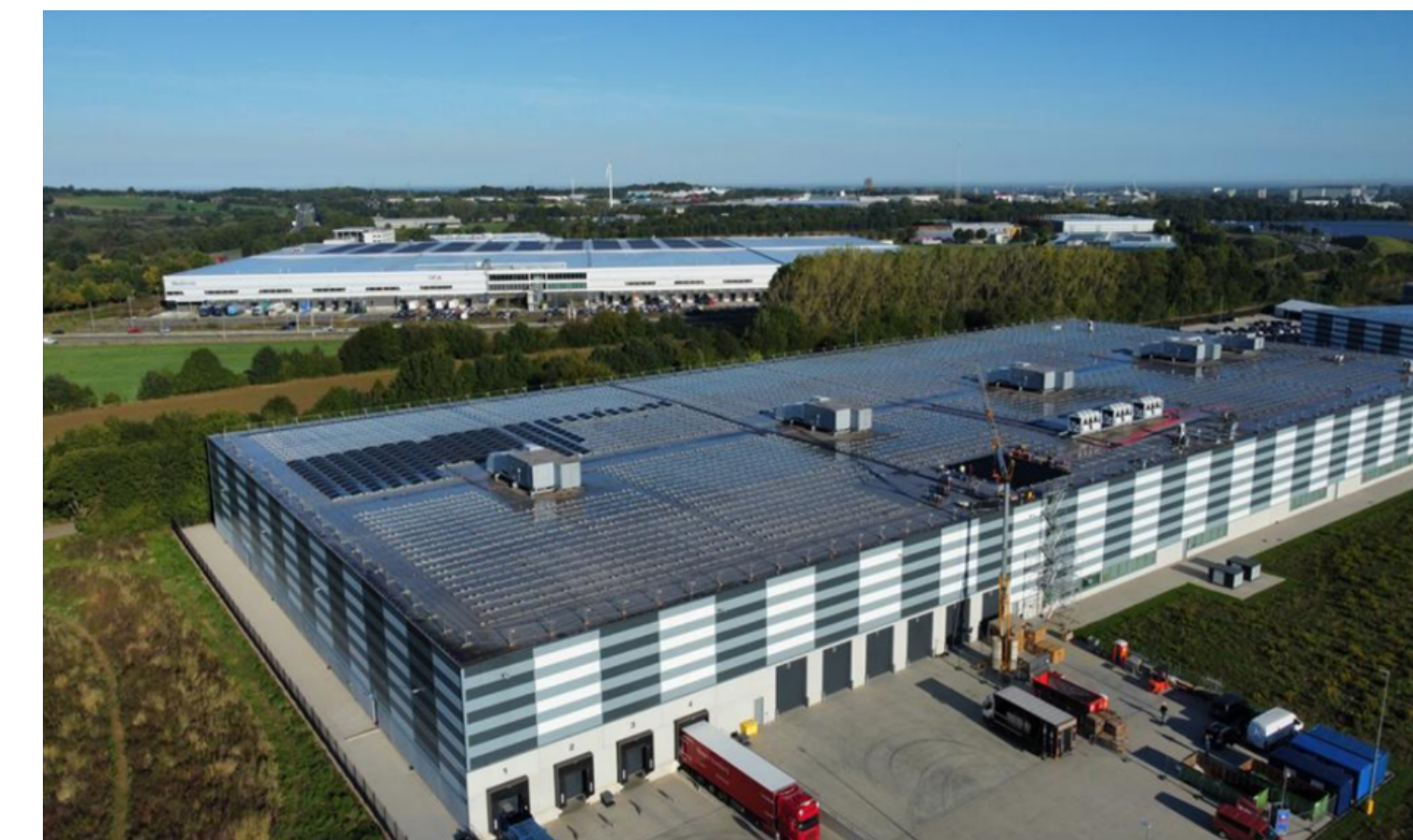
DocMorris' new Distribution Centre 2 in Heerlen, the Netherlands
