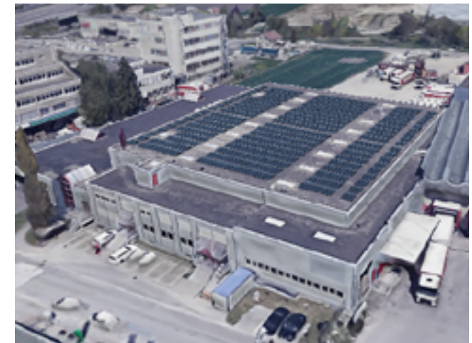
Large photovoltaic system in Dietlikon, UBS AST-KIS 1)
