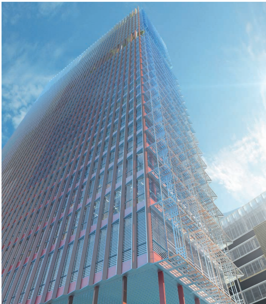
32-storey office building in Marseille in conformity with environmental certifications such as HQE Excellent and Leed Gold © AJN
