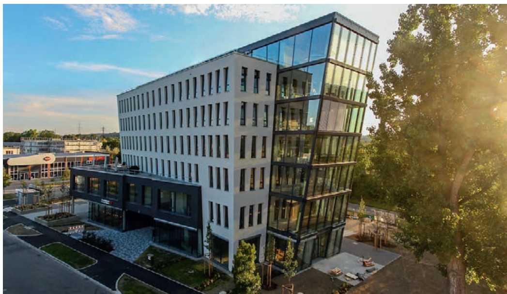
The LEED Platinum pre-certified office building in Augsburg is part of a Corpus Sireo real estate fund
