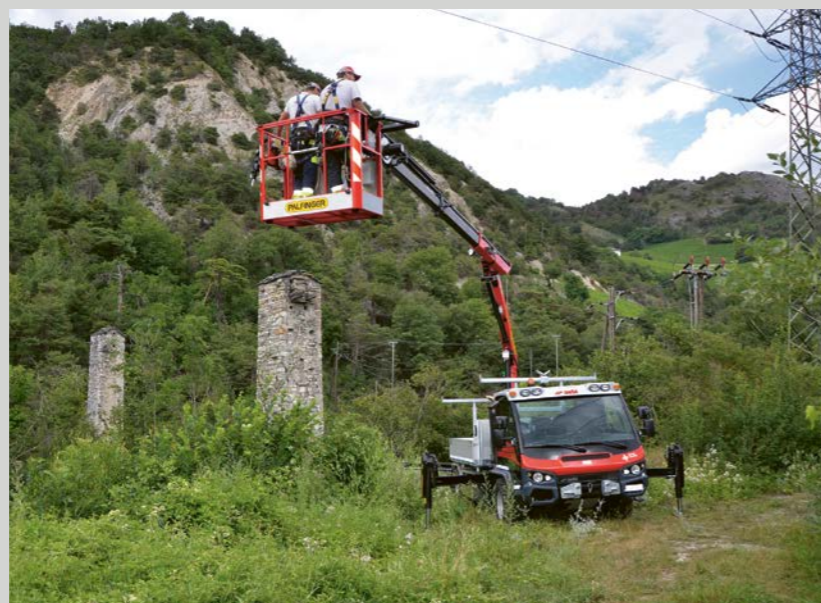
Aebi at work for the energie company ReLL in Susten (CH)
