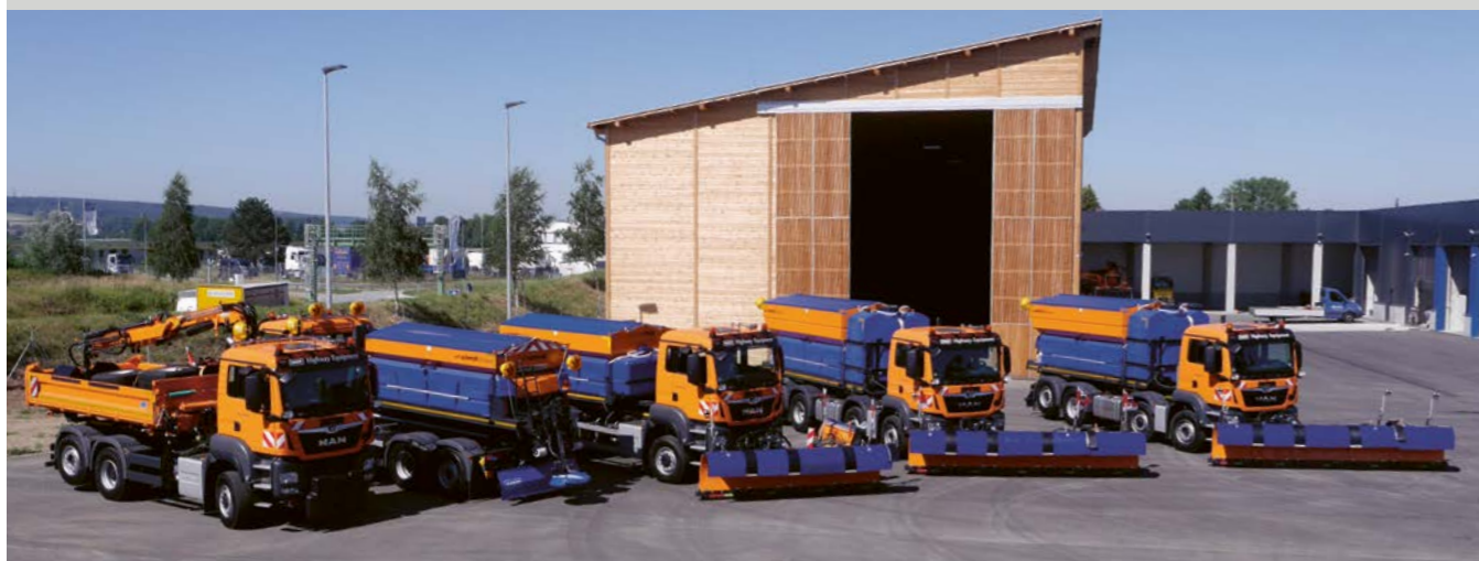
The fleet at the new motorway depot in Ampfling
