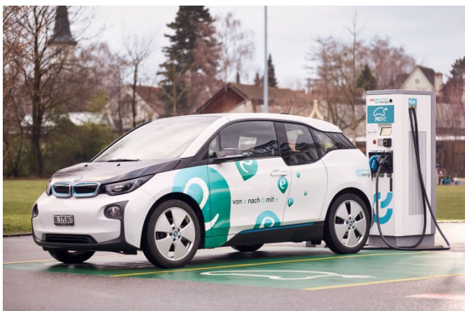
MOVE-Ladestation in Therwil
