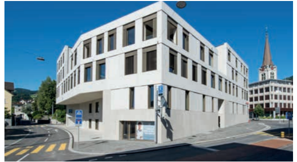
Altstätten, Churerstrasse 1a, 1b, 1c
