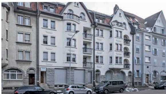
St. Gallen, Oststrasse 18, 20
